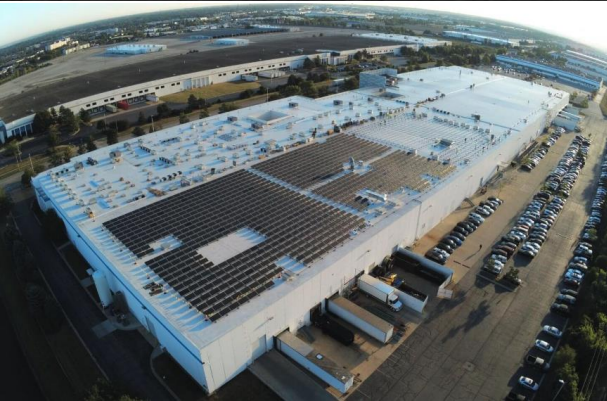
G&W Electric microgrid solution - Illinois, US. – 8MWh
